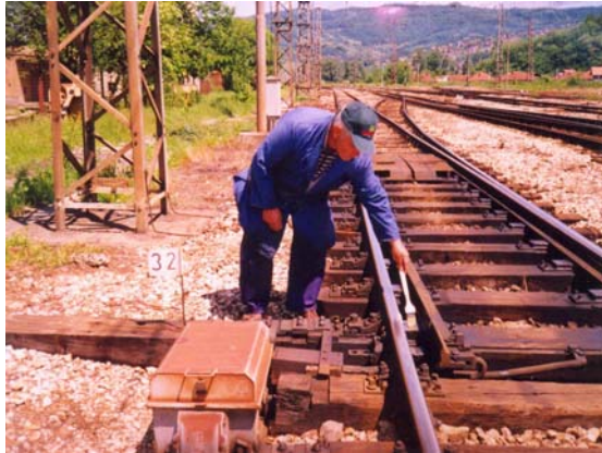
Figure 9: Lubrication of the pad of the track by a brush
