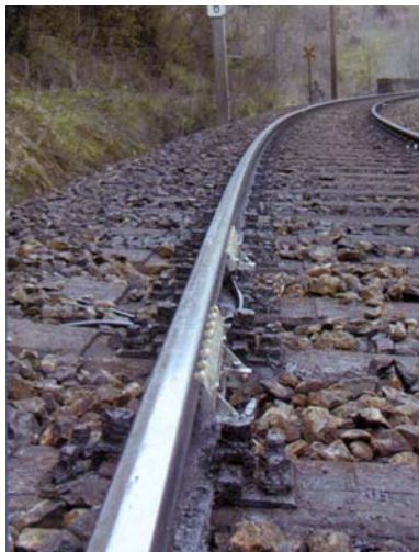
Figure 5: Lubricating device tied to the tracks
