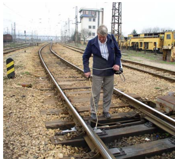
Figure 8: Lubrication of the pads of the track by grease gun
