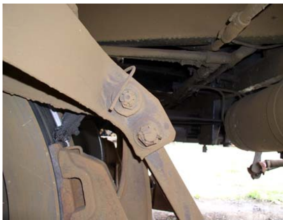
Figure 6: Lubricating device tied to the locomotive
