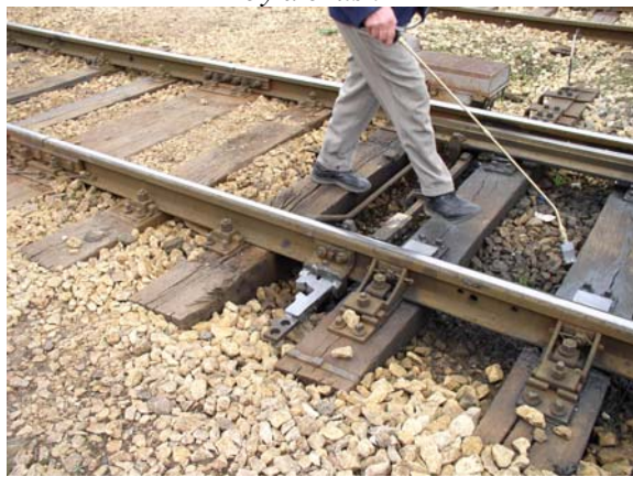
Figure 10: Movable parts of the switch that are lubricated
